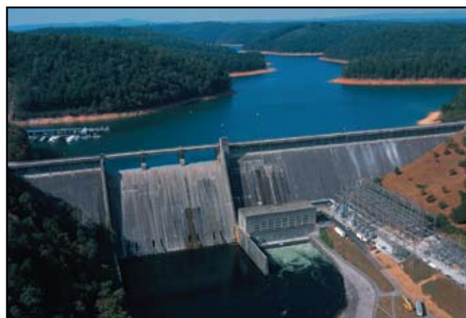
Norris Dam on the Clinch River, Tennessee, the first large dam built by the Tennessee Valley Authority in 1936. Large dams fragment populations, impede migration of fishes, and are points of introduction for many nonindigenous fishes.
