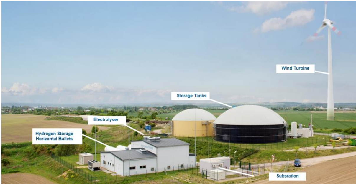
Figure 6-3: Enertrag Germany's Hybridkraftwerk
