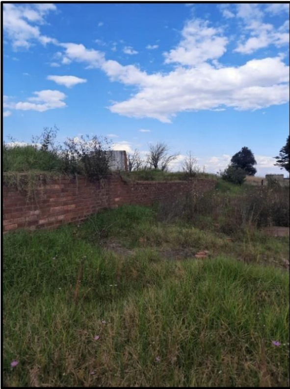
Figure 7-38: Brick structures at Waypoint 097
