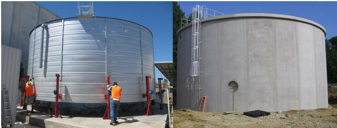
Figure 6-11: Typical water reservoir (left - concrete, right – steel)
