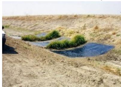
Vetiver filter strips installed on a drain on a cotton farm in Australia
