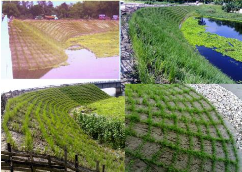
Doria Bridge approach , before and after vetiver planting , note grid pattern
