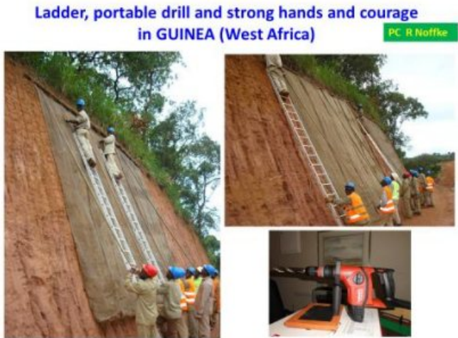
Hydraulic borer used to plant vetiver on slope with very hard subsoil
