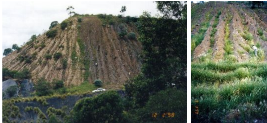
This coal mine waste dump was barren for 50 years. Before and after vetiver planting for erosion control
