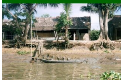
Bank erosion caused by waves from river traffic erosion
