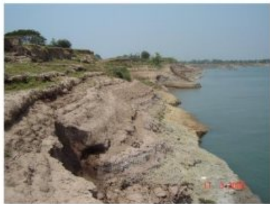
Erosion on the Mekong bank
