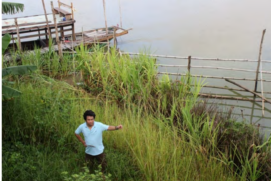
Figure 16. Co De planting for riverbank stabilization
