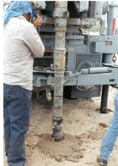
Auger boring for a Monitoring Well
