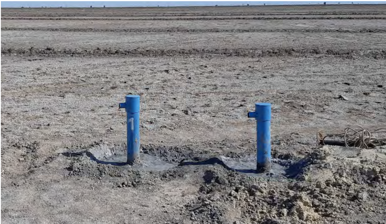
Fig. 36. Groundwater table monitoring wells, GKH-6, installed in July 2019, Sudochie-Adjibay section
