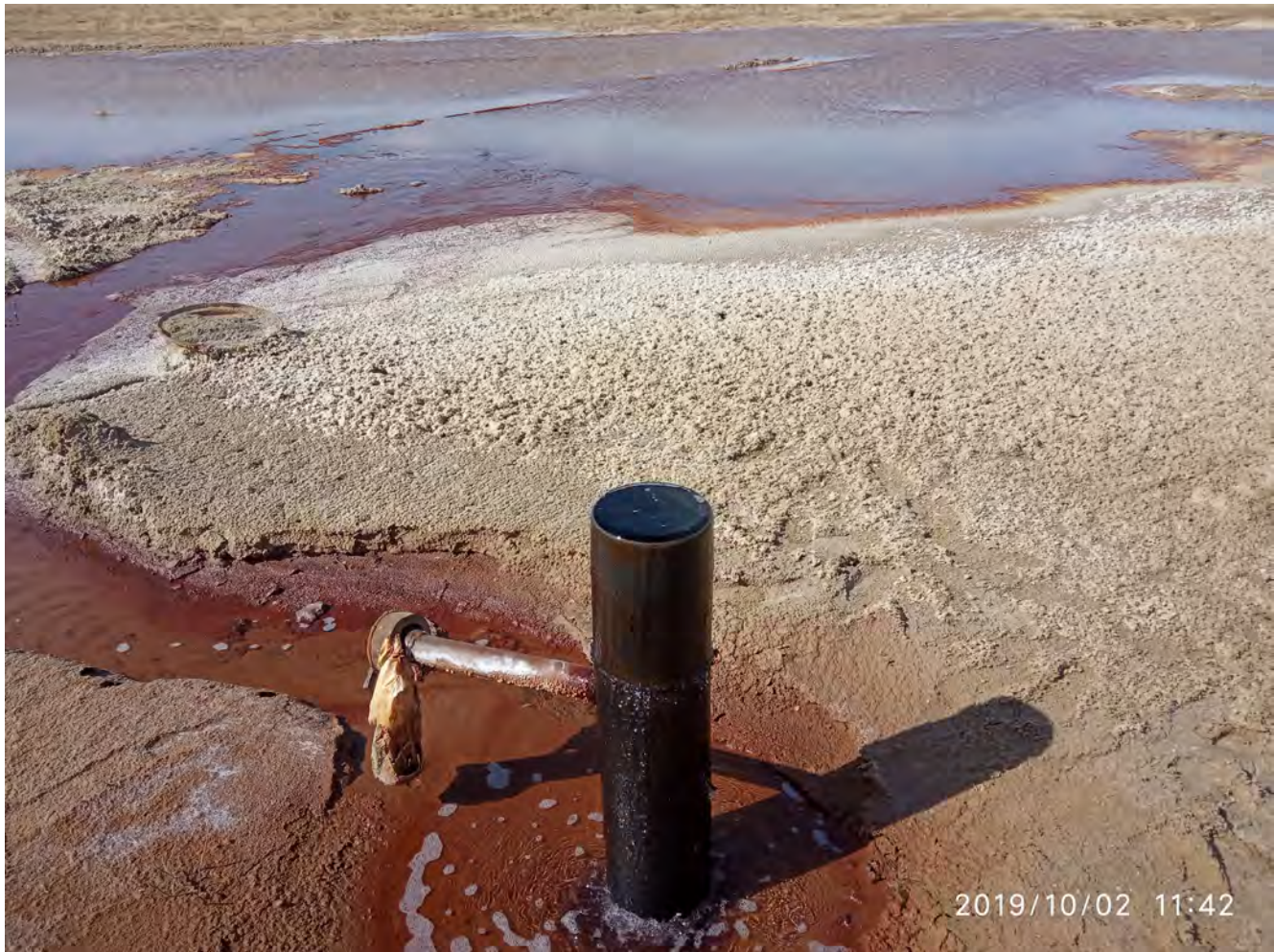
Fig. 38. Self-discharging wells on the road to Vozrojdenie (Ascension)
