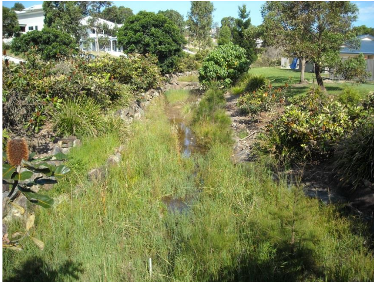
Plate 15 - Drainage line managed by NRMU as an extension of Zone 4 The vegetation is naturally regenerating native grasses and sedges
