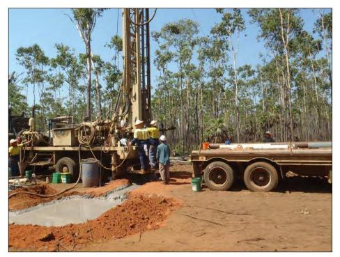
Figure 3: Water Resources drilling operation on Bathurst Island
