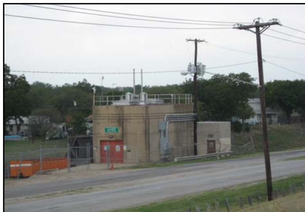
Figure 3-3 Pavaho Pumping Plant
