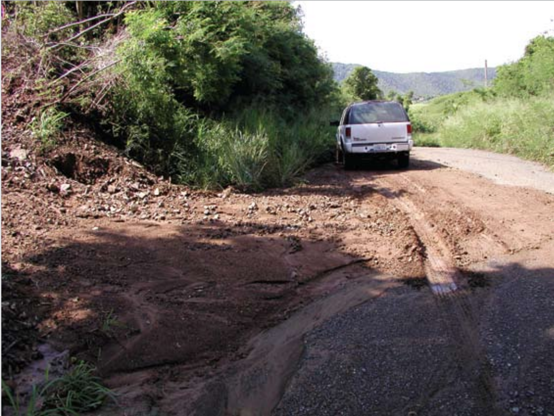
Uncontrolled soil erosion resulting from construction damages both terrestrial and marine ecosystems. (photo by Tom Brandeis)
