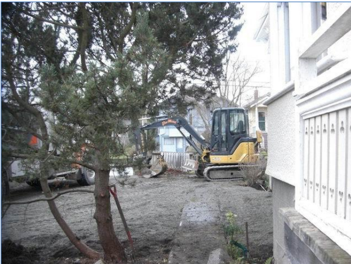
Left: The excavator on site
