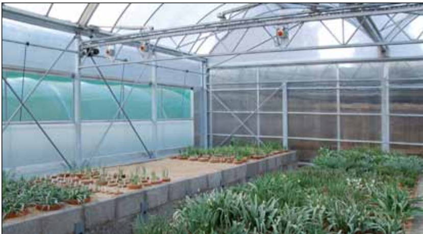
85 - Inside the first Rovero polytunnel in Scotland
