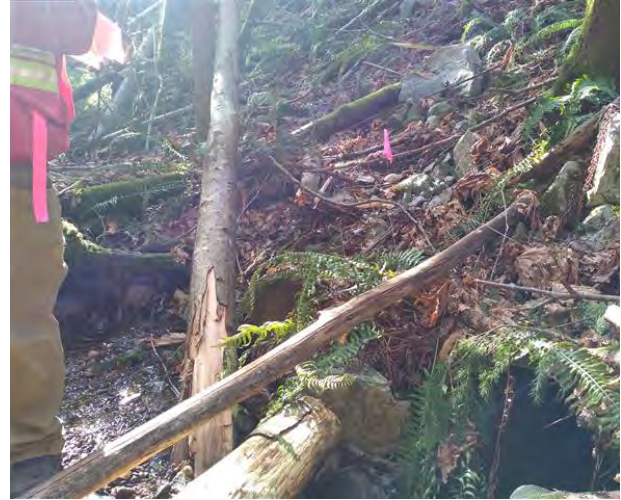
Photo 71: Culverts leading under the railway line in Watercourse 1. February 22, 2019.
