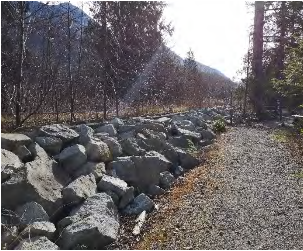
Photo 89: Trail and retaining wall located adjacent to Furry Creek foreshore. February 7, 2019.
