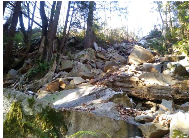
Photo 50: Looking upstream at large boulders in lower section of Middle Creek Tributary 1. February 5, 2019.
