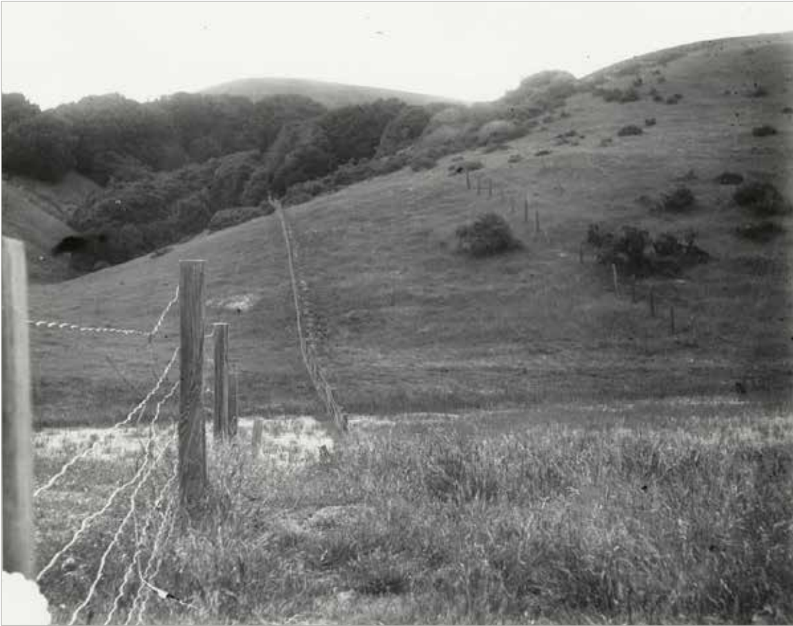
Figure 1.4. This photograph, taken shortly after the 1906 earthquake, shows the offset in a fence between San Andreas and Lower Crystal Springs reservoirs resulting from movement of the San Andreas Fault. (BANC PIC 1957007 Ser. 2 :087, courtesy The Bancroft Library, UC Berkeley)
