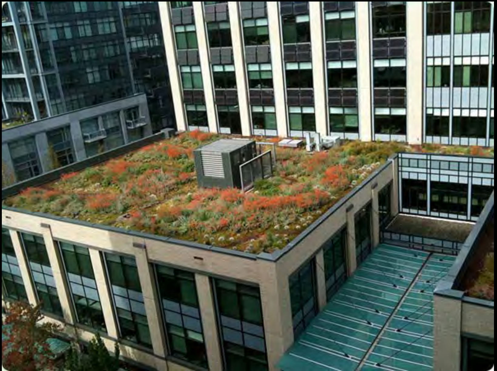
M Financial Building green roof in Portland
