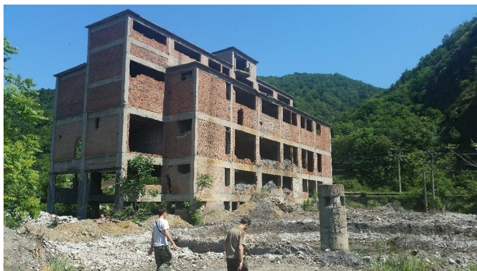
Figure 201 Demolished industrial site, Cozla, Caraș-Severin County (foto: Iulia Miu)
