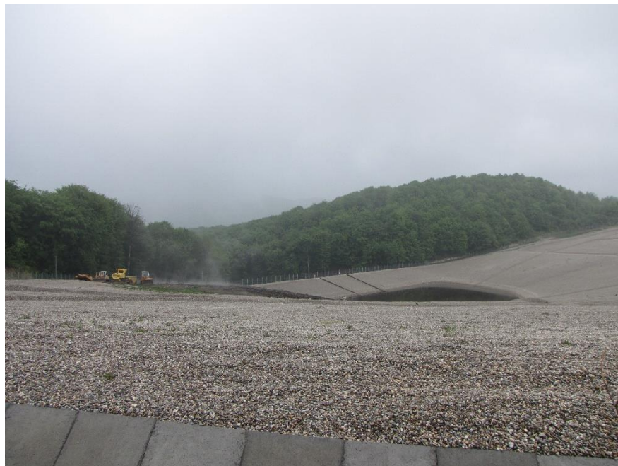
Figure 225 Waste storage, Râmnicu Vâlcea, Vâlcea County (foto: Iulia Miu)
