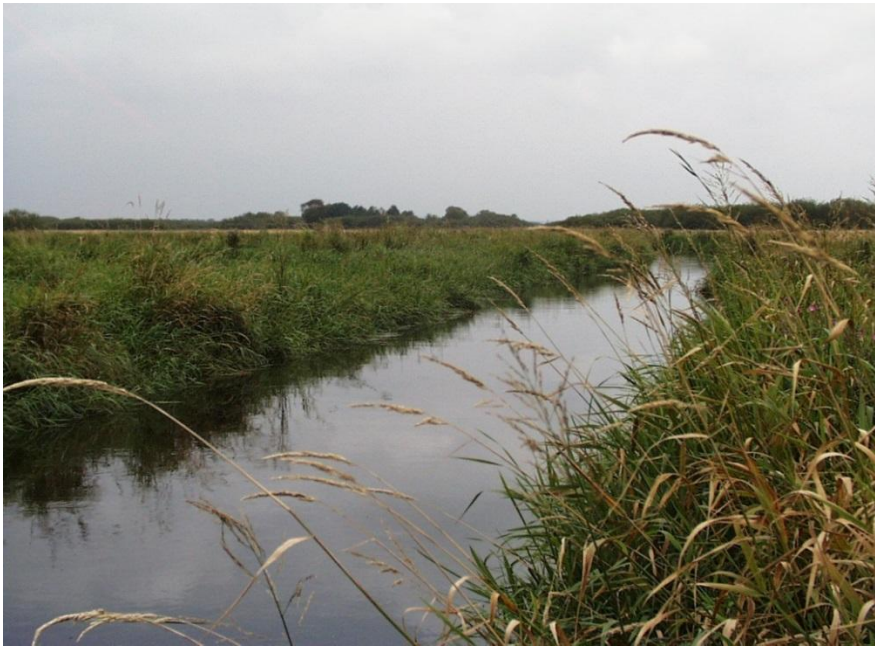
Figure 3.1 Part of Skals å situated in Jutland, Denmark. This section has been straightened and deepened to improve drainage from adjacent areas.
