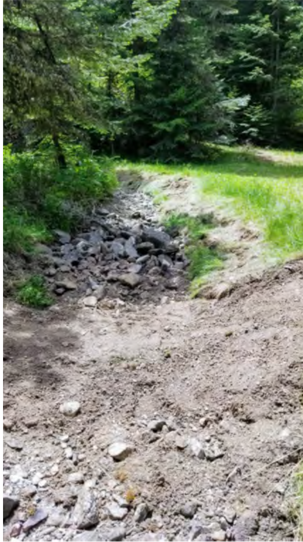
Photo 7: Decommissioned south tailrace channel – lower crossing
