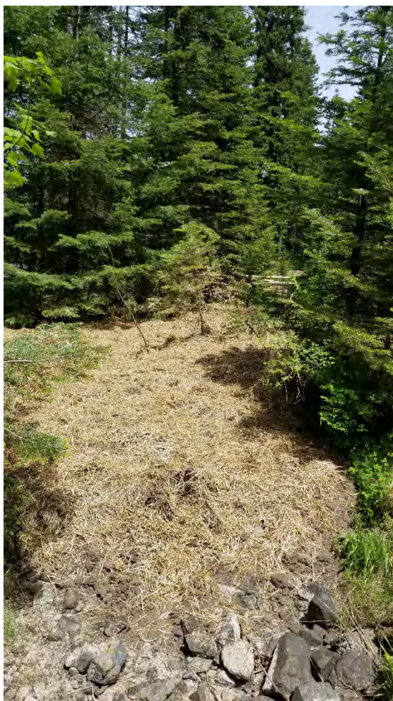
Photo 6: Decommissioned south tailrace channel – seeded and mulched
