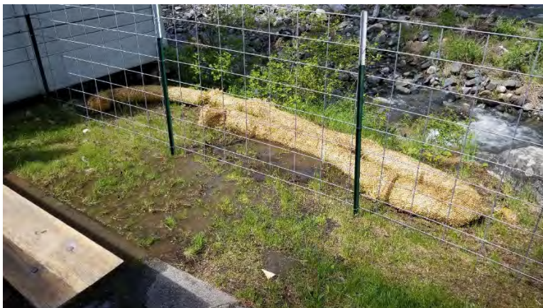
Photo 2: Active discharge and wattle placement to slow runoff into river
