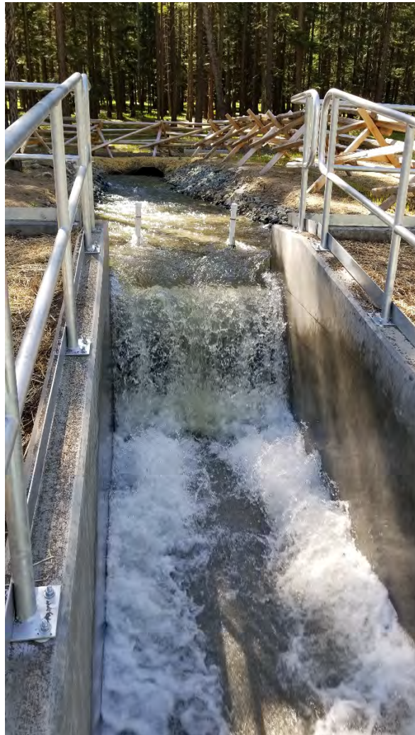
Photo 3: Weir and box flume at tailrace outlet (June 5, 2020)
