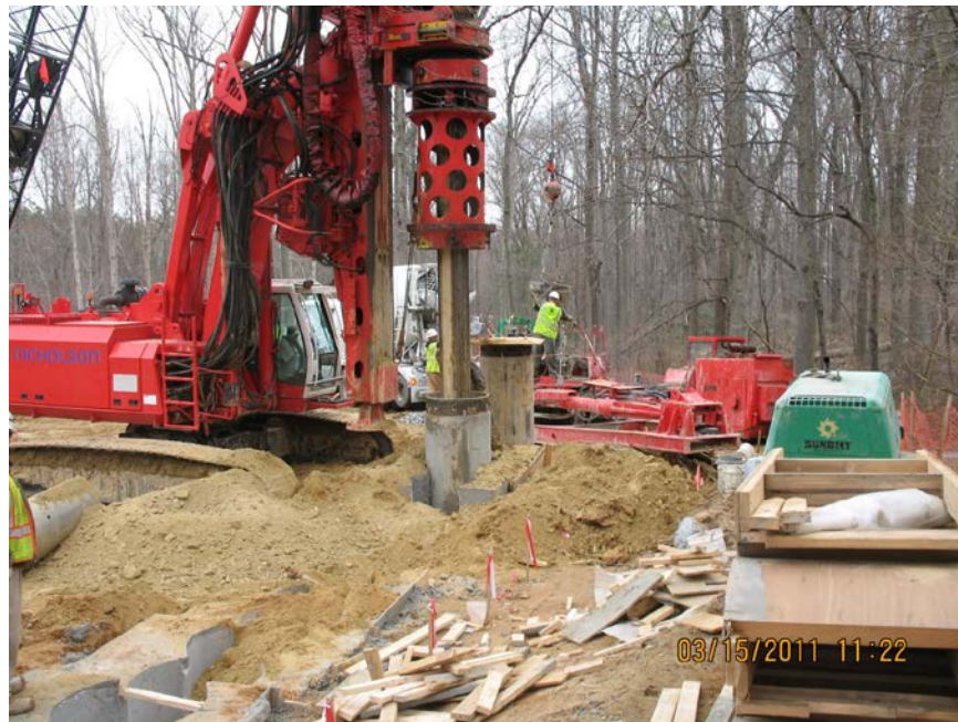
Figure 8. Installation of secant pile wall.
