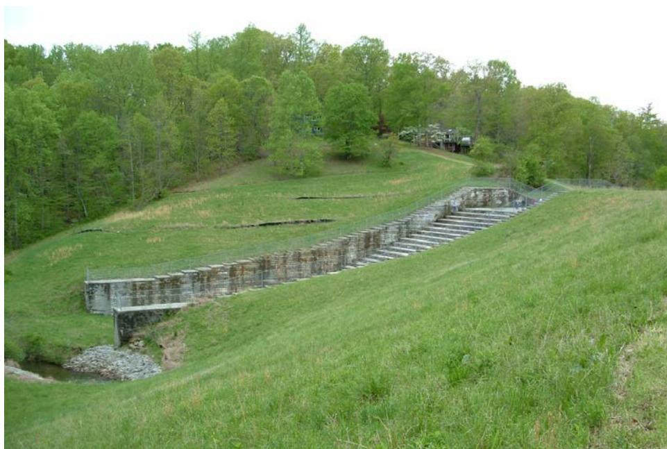
Figure 11. The RCC auxiliary spillway at White Oak dam, Madison County.
