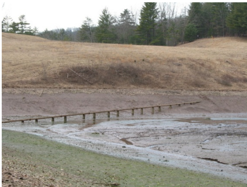
Figure 4. Sewer line observed when lake is drained.
