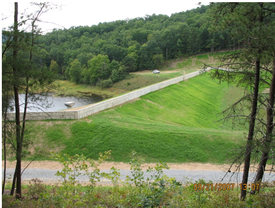
Figure 10. Parapet wall on top of a dam.
