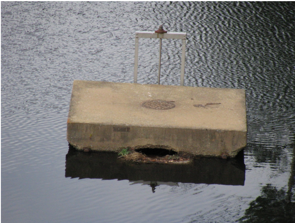
Figure 3. Principal spillway riser at Todd Lake (October 2010).
