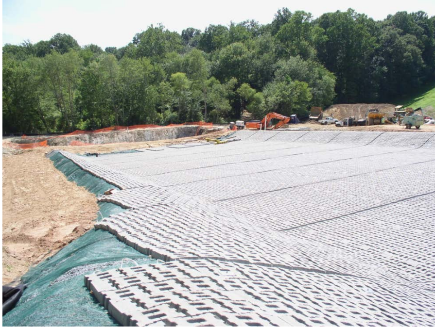
Figure 9. Installation of ACBs.
