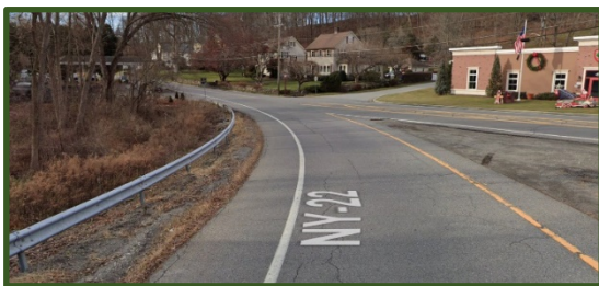
Entering hamlet near Croton Falls Fire House
