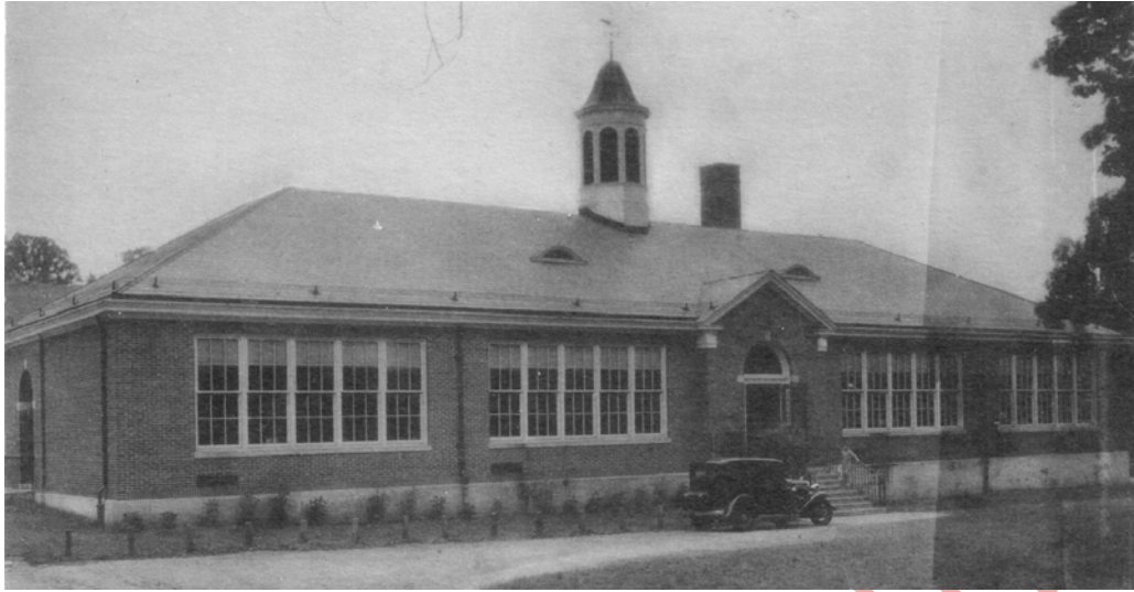
16. 3 Owens Road , 1.1-1713-3. Constructed 1926. Originally Rural School No.2 for the town. Simple Colonial Revival style school designed by architects Knappe and Morris. Photos 1928, 1986 – little has changed. Slate roof still intact. First photo Curtis postcard, second WC 1986.
