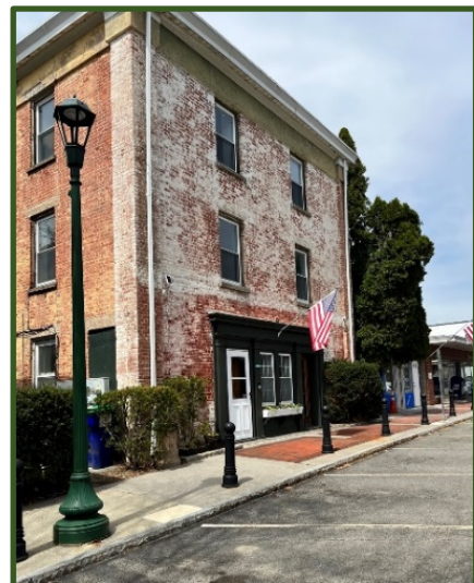
4 Front Street Colley Group offices
