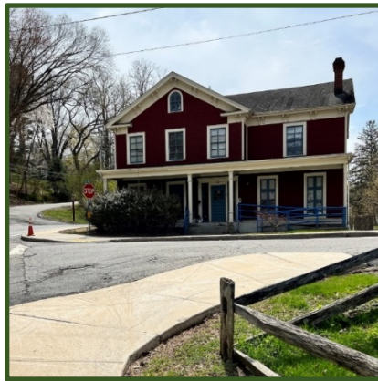
2 East Cross Street – Circa 1860 Three Apartment Units
