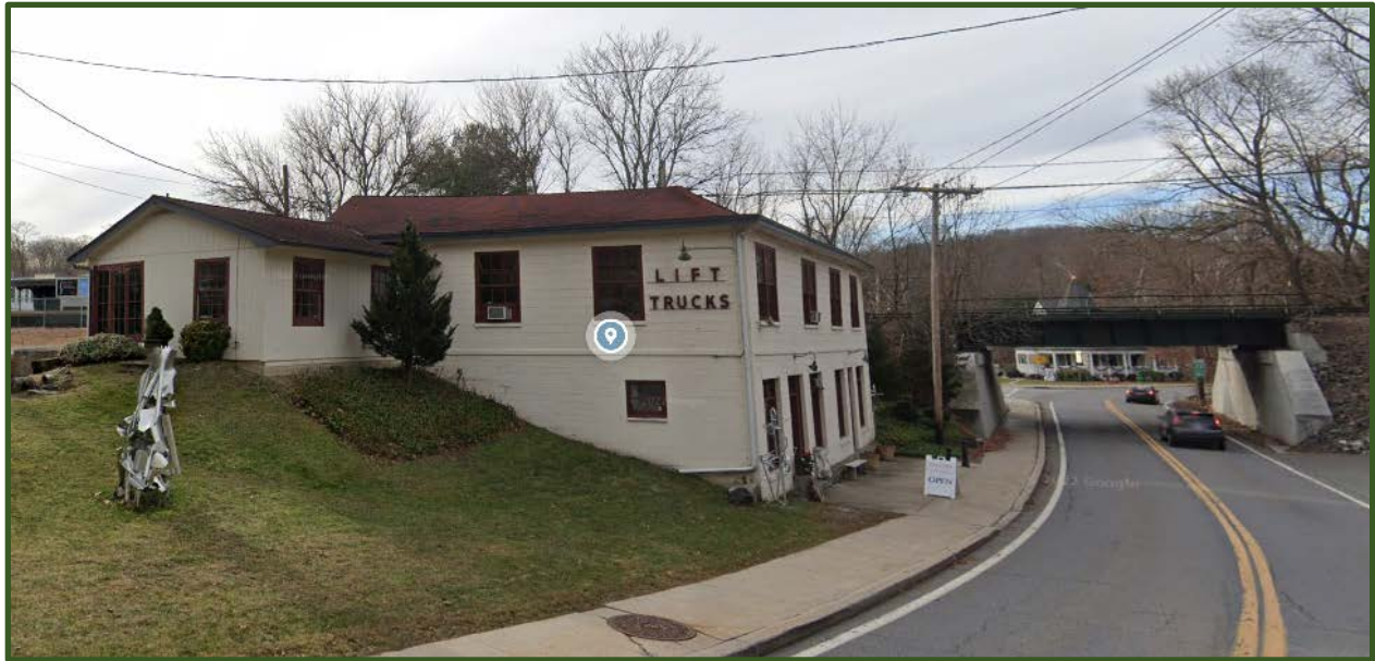
3 East Cross Street – Circa 1922 – Lift Trucks transformed to art studio and workshop
