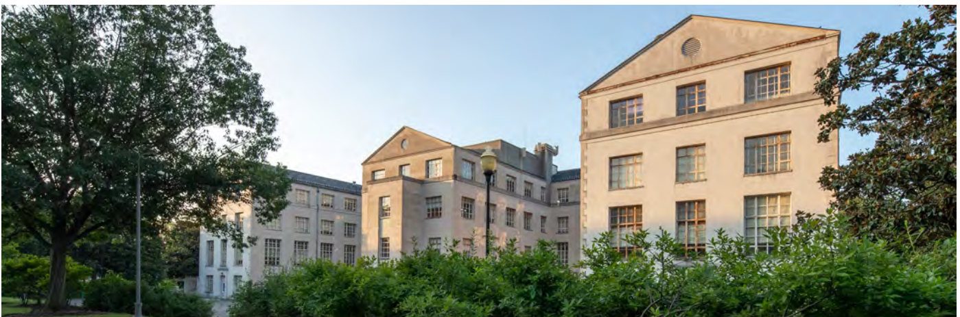
Figure 3.15: North elevation, FRB-East Building.
