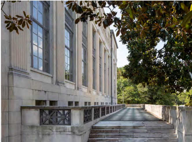
Figure 3.17: View of building terrace, FRB-East Building.
