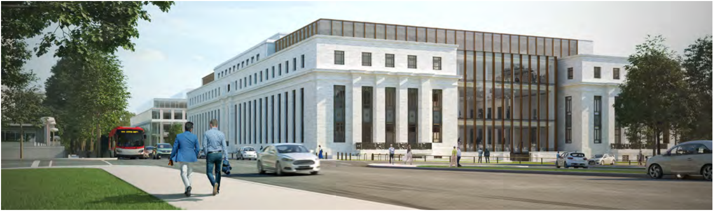
Figure 2.7: View of Eccles Building and proposed infill looking southeast from C Street showing 21st Street elevation.
