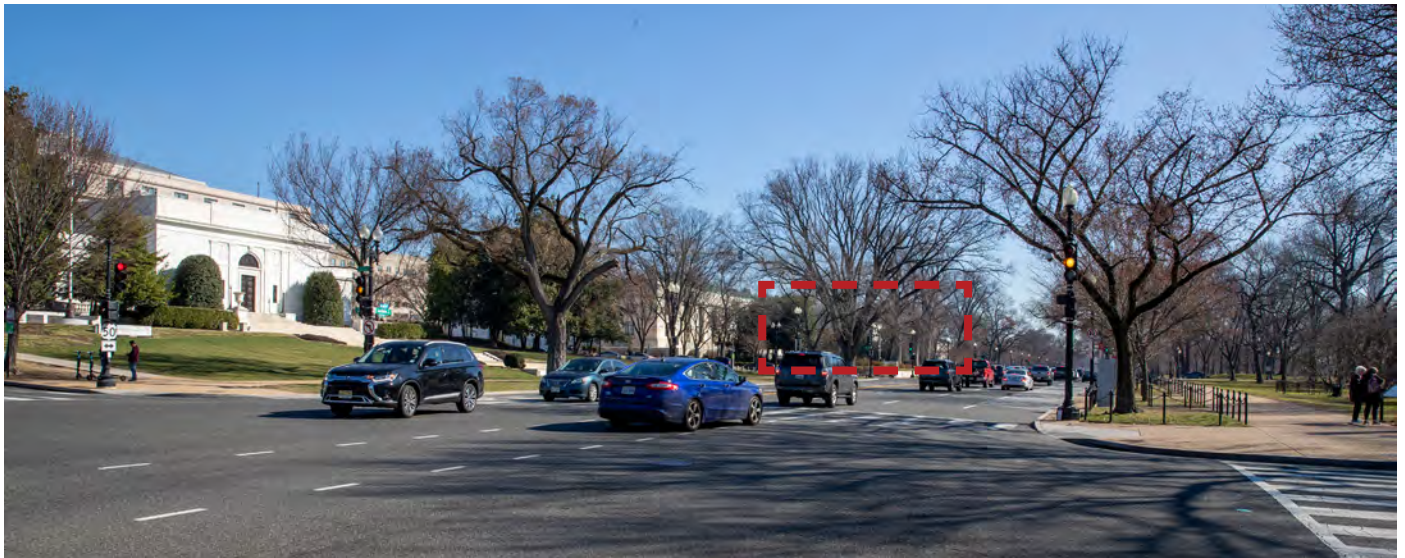
Figure 4.30: Existing view looking northeast along Constitution avenue from 23rd Street toward project area.
