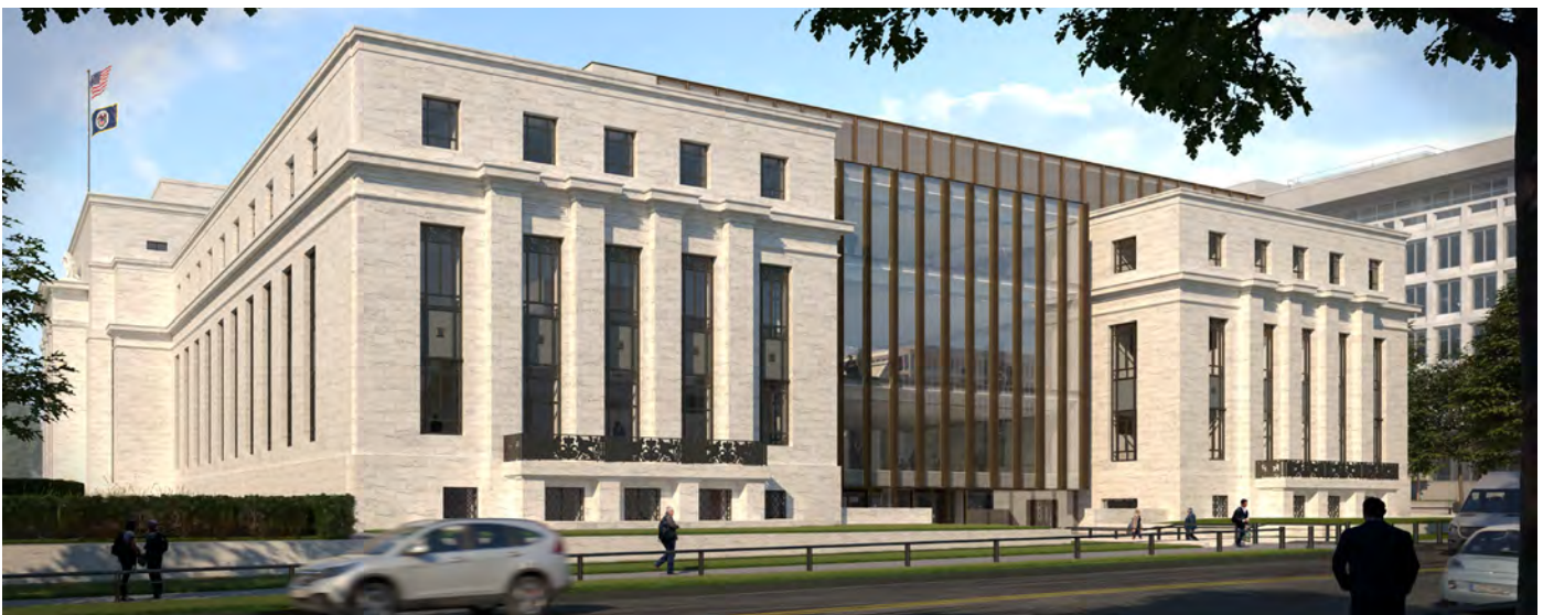
Figure 2.9: View of Eccles Building and proposed infill looking northwest showing 20th Street elevation.
