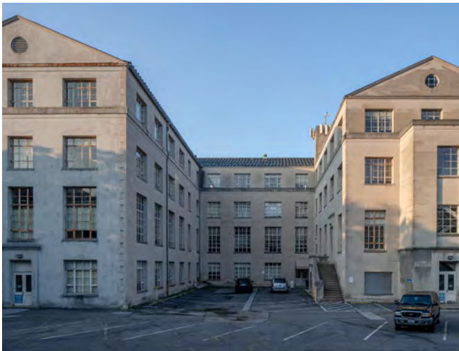
Figure 3.18: North Elevation, center wing, FRB-East Building.
