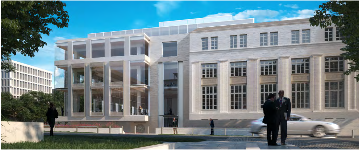
Figure 2.21: Alternative 2: View of FRB-East Building and proposed addition looking northeast toward main entrance.
