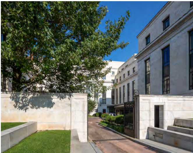
Figure 3.8: Site walls of east courtyard.
