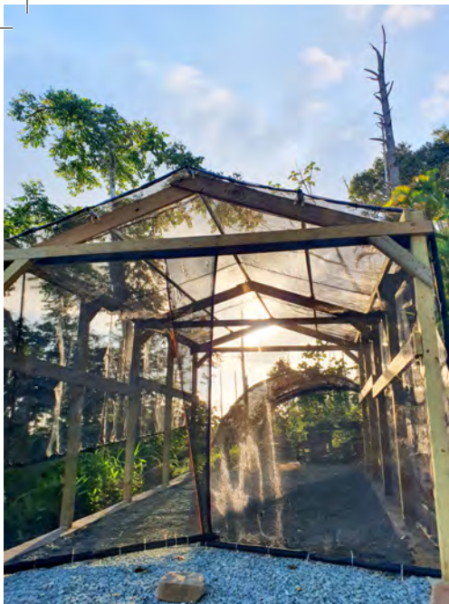
The new nursery takes shape in Puerto Rico.
