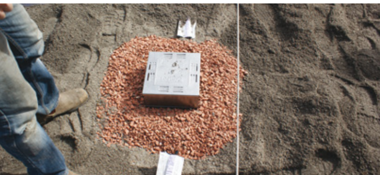
Non-vegetated zone around hard infrastructure on a roof
