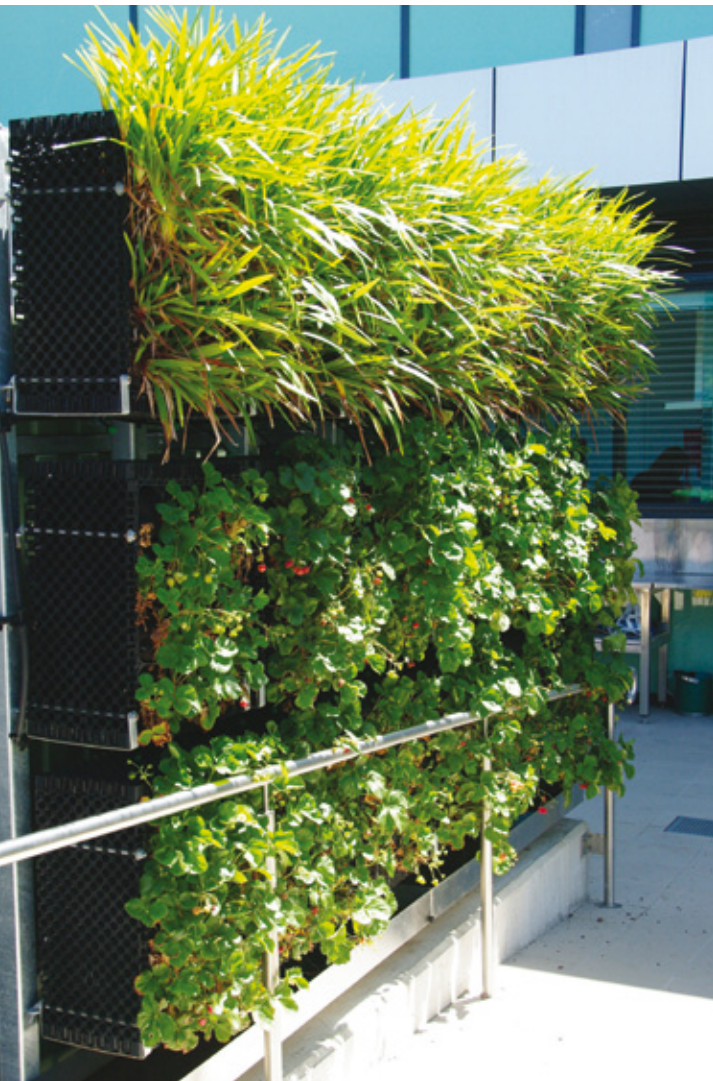
This green wall on the roof of a health care centre in Marion, South Australia, incorporates an inbuilt water tank to provide water supply and structural integrity for double sided modular wall systems, with plantings including strawberries and herbs. Image: Fifth Creek Studio
