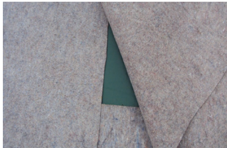
A protection mat is laid to protect the waterproofing layer on a green roof
