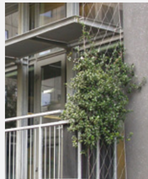
Figure 23. Support structures for green facades grown with twining climbers
