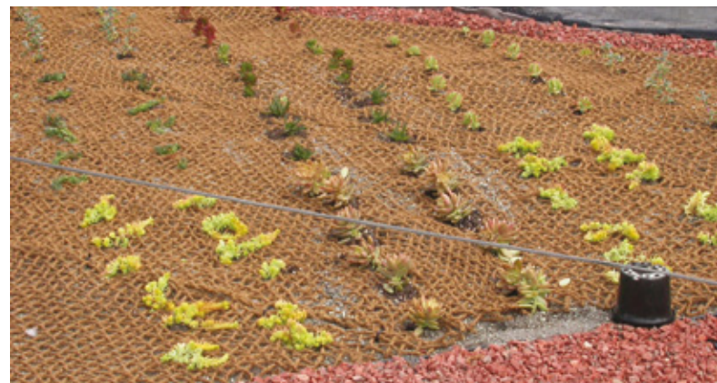
Roof A was planted with a mix of Australian and exotic herbaceous and succulent plant species
