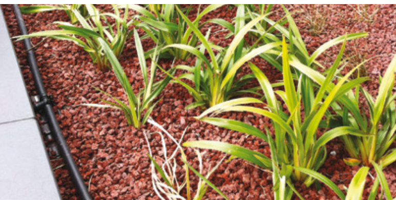
This green roof at the Peter Doherty Institute, Grattan Street, Parkville, functions as a grey water treatment system. Image: Eco Harvest
