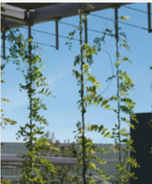
Figure 23. Support structures for green facades grown with twining climbers
