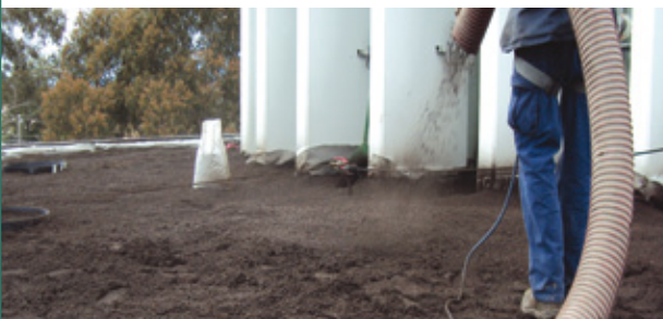
Substrate was blown onto the green roof in the City of Monash, Glen Waverley. Image Junglefy
