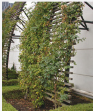
Figure 23. Support structures for green facades grown with twining climbers
