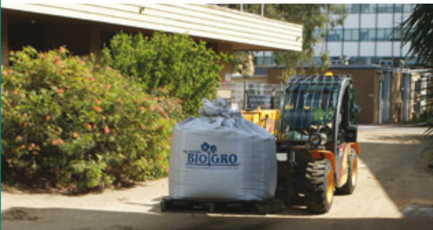
Bulker bags of substrate moved around the site, at ground level, prior to being lifted by crane at the demonstration roof at The University of Melbourne's Burnley campus
