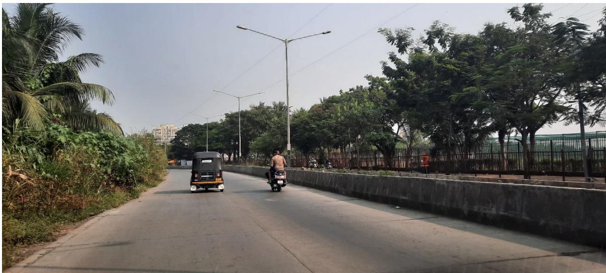
Scope for median plantation on Uttan Road, Bhaindar West
