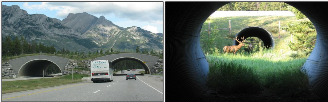
Wildlife overpass and underpass at Banff National Park in Alberta, Canada. Photo credit: flickr/Roswellgirl, Source: http://www.smithsonianmag.com
