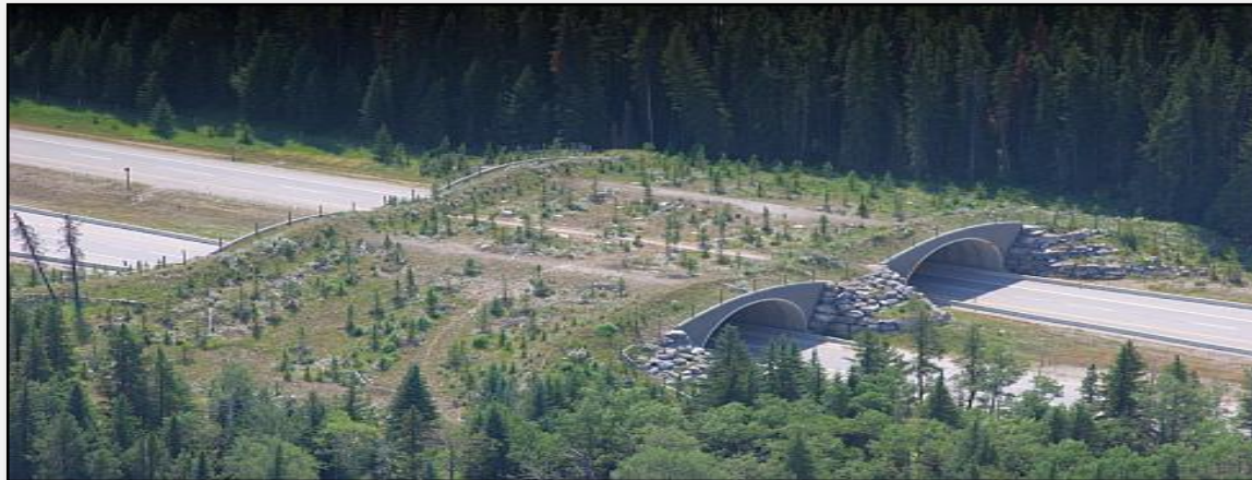
The overpass or “Ecoduct” constructed over Trans-Canada Highway at Banff National Park, Canada. Image source: http://highwaywilding.org
