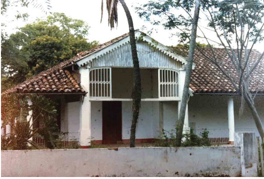
FIGURE 61. Hassler's Villa Mon Repos in 1987, two years before being demolished. Photograph by Lorenzo Ramella.
