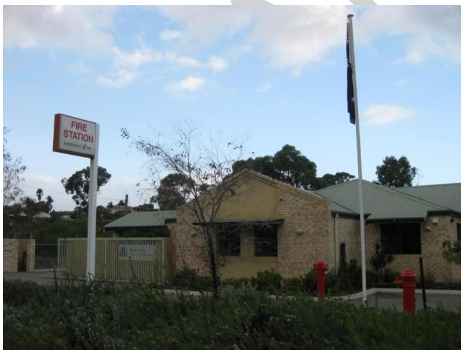
Figure 30: Dun Craig Fire Station
