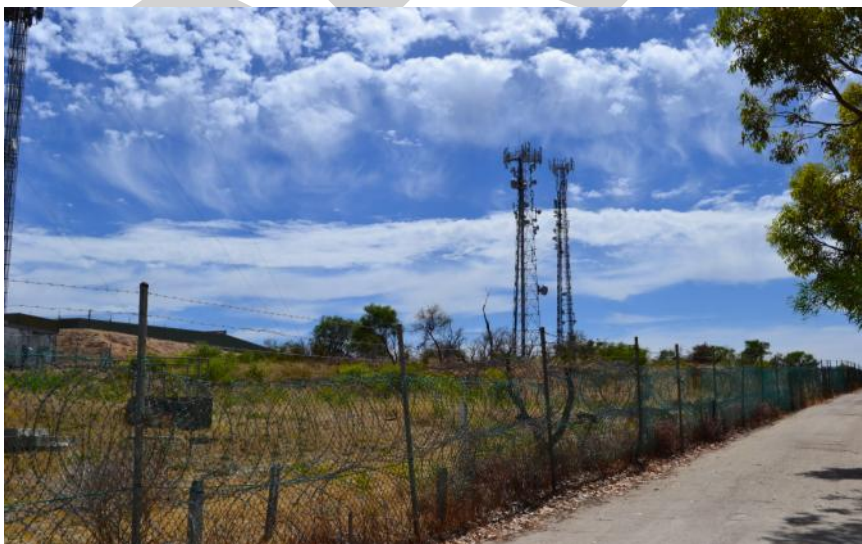
Figure 29: Water Supply and Telecommunications Facility
