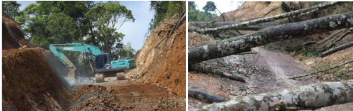
Figure 21d. Road construction along the Lao-Vietnam Border and TL clearance
