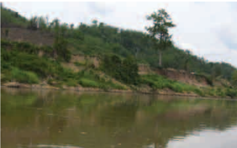
Plate 3.7. Removal of Strand and terrestrial vegetation along the Mekong River has resulted in the collapse of many embankments. Opposite Ban Donmen,
