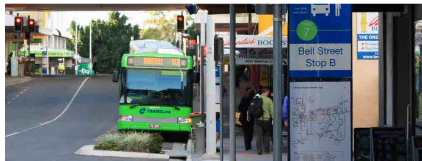
Bus indent bay and associated infrastructure. Bell Street, Ipswich Central.
