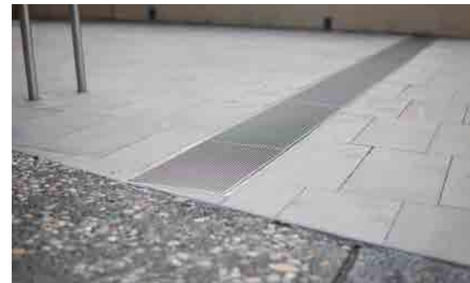
Stone paving and coloured exposed aggregate concrete, Ellenborough Street, Ipswich
