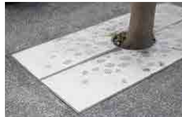
Custom tree grates, Ipswich Central
