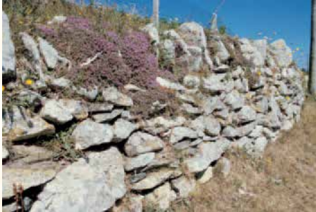
Retaining wall (L.Lysaght)
