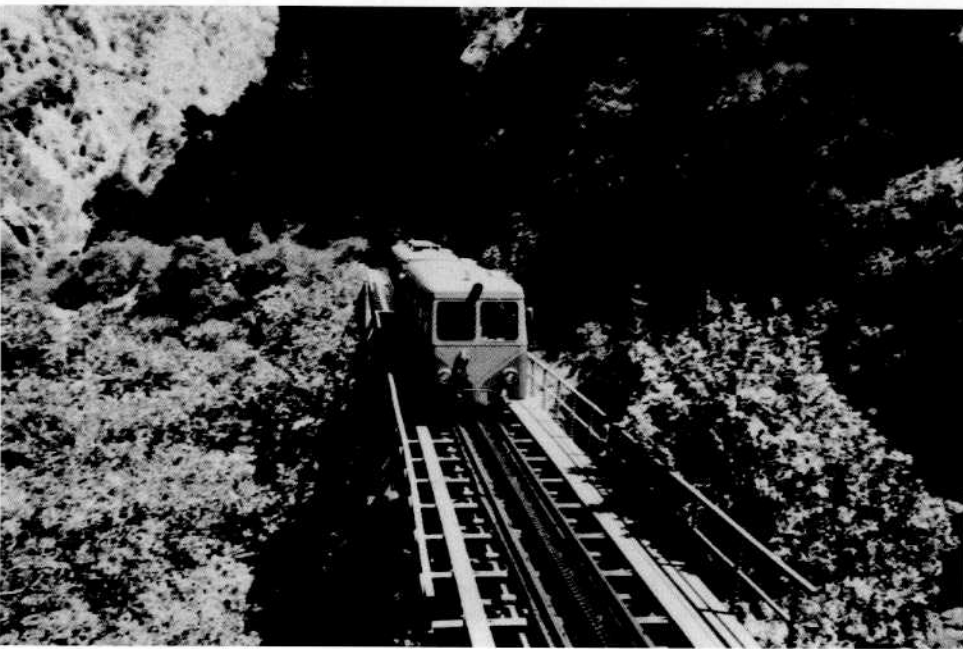
Fig. 4. The rack railway which crosses the gorge over iron brigdes.
