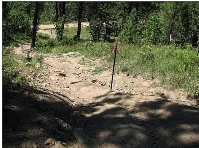
Figure 15. Example of a fence built to block ATVs from shortcutting roads
