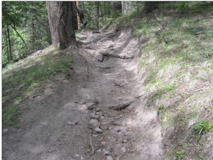
Figure 50. A system trail that is incised, forming a channel through which water flows. As the water flows, it pulls more soil down with it. Even without motorized use, this system trail is not likely to revegetate on its own within 15 years.
