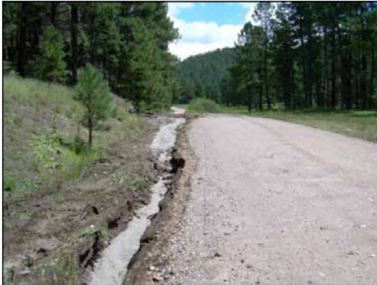
Figure 44. An example of how roads alter the patterns of runoff in a watershed. Water normally flows down a hill in a sheet. Here, the bar ditch adjacent to the road intercepts the water, concentrating it in one fast channel, which is downcutting and carrying sediment. From an engineering perspective, the bar ditch is doing its job: keeping water off the road.
