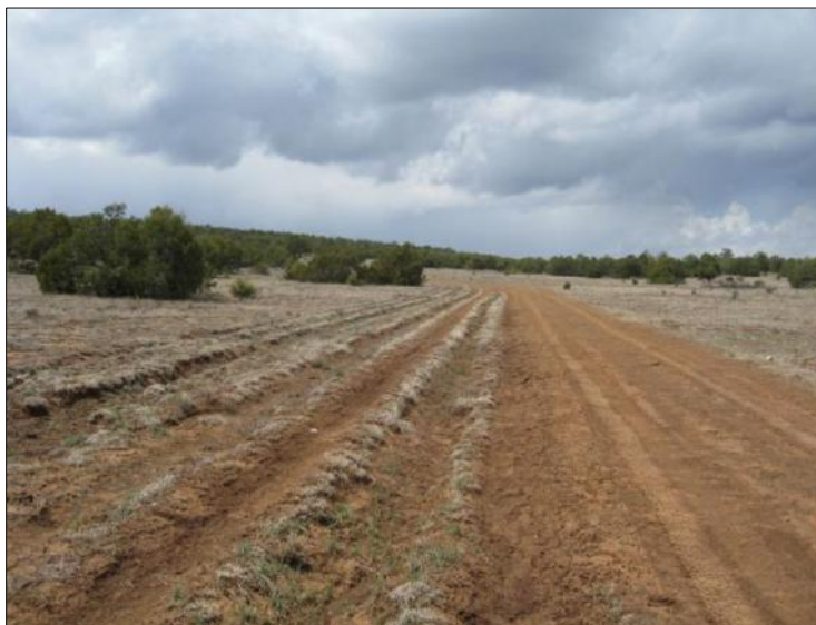
Figure 46. Photo illustrating the concept of braiding. When the main road is muddy, people drive to the left, widening the road.
