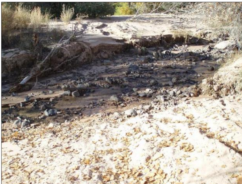
Figure 42. Road leading to private property that is causing damage to the stream and riparian area
