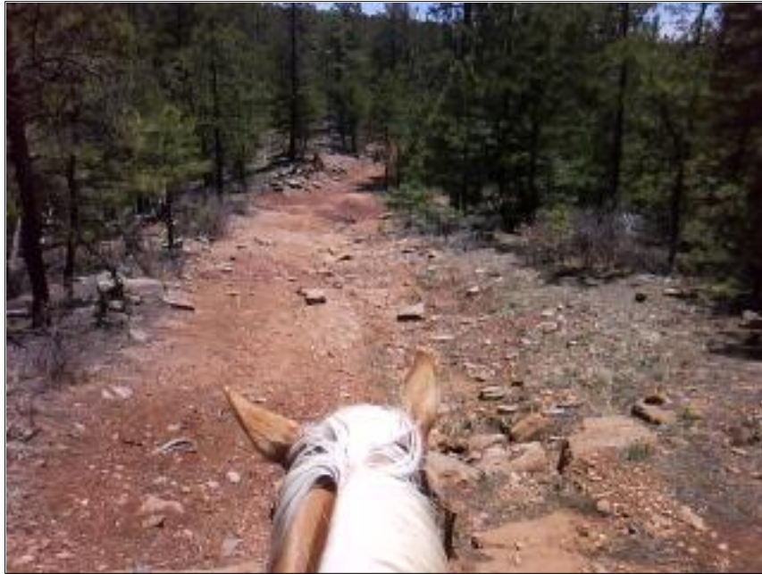
Figure 49. A National Forest System road that has been closed to use, but continues to erode. There is an erosion channel starting above the horse's right ear and leading to the top of the photo.
