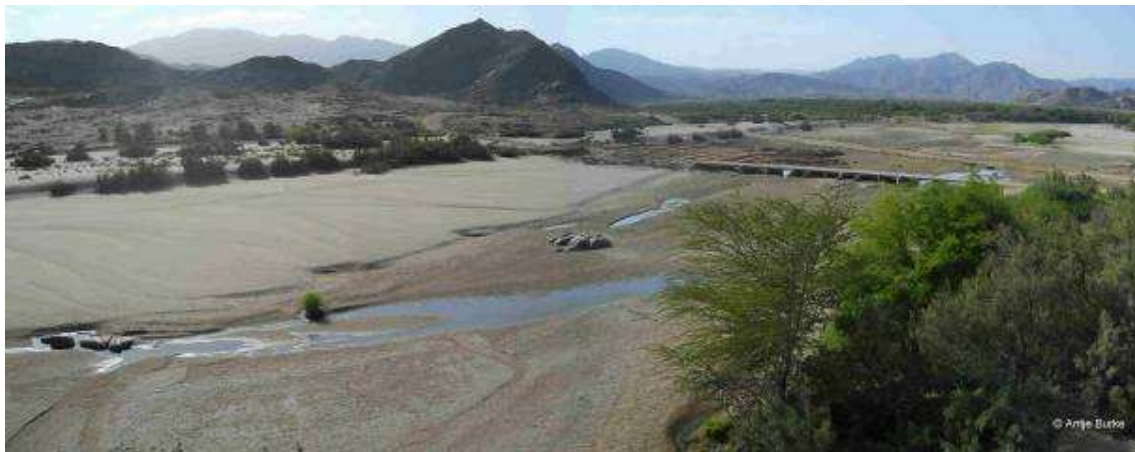
The bridge over the Fish river near the Orange river confluence is washed out regularly by flash floods.
