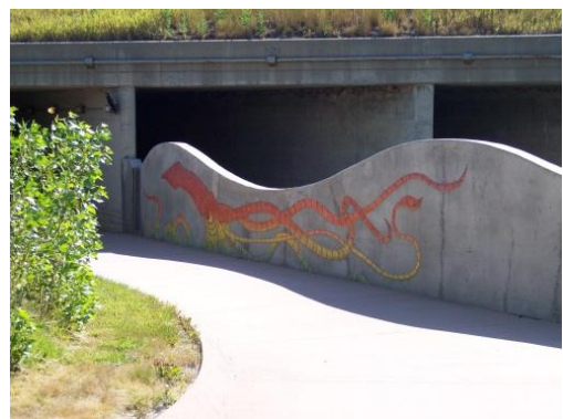
Mario Echevarria's Trail underpass APP Project
