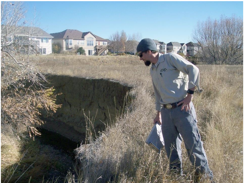
Inspecting Mail Creek social trail for hazards
