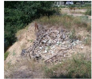
Bank debris accumulation along the Inlet Ditch
