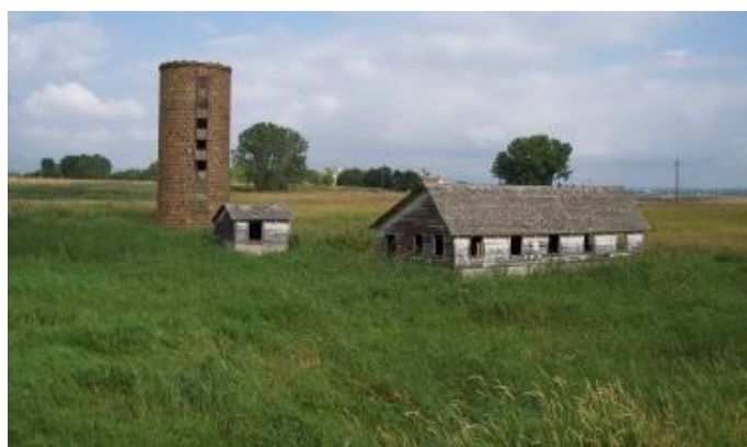
Historic silo and outbuildings
