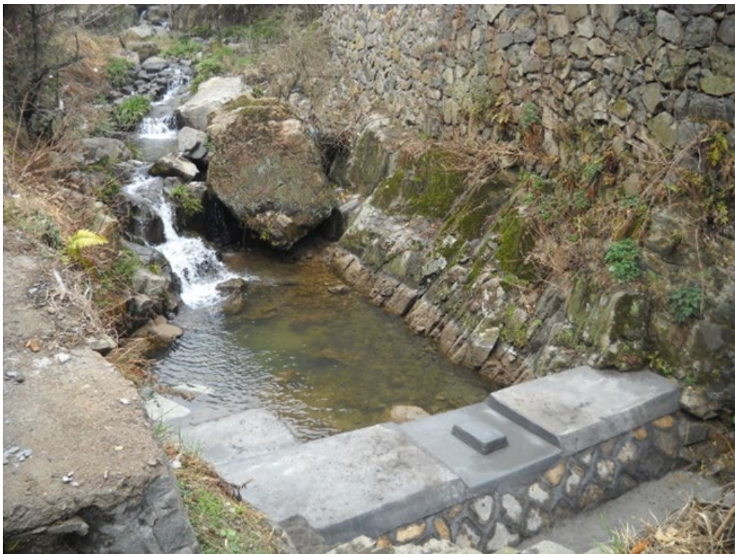
Figure 43 Check dams in mountains
