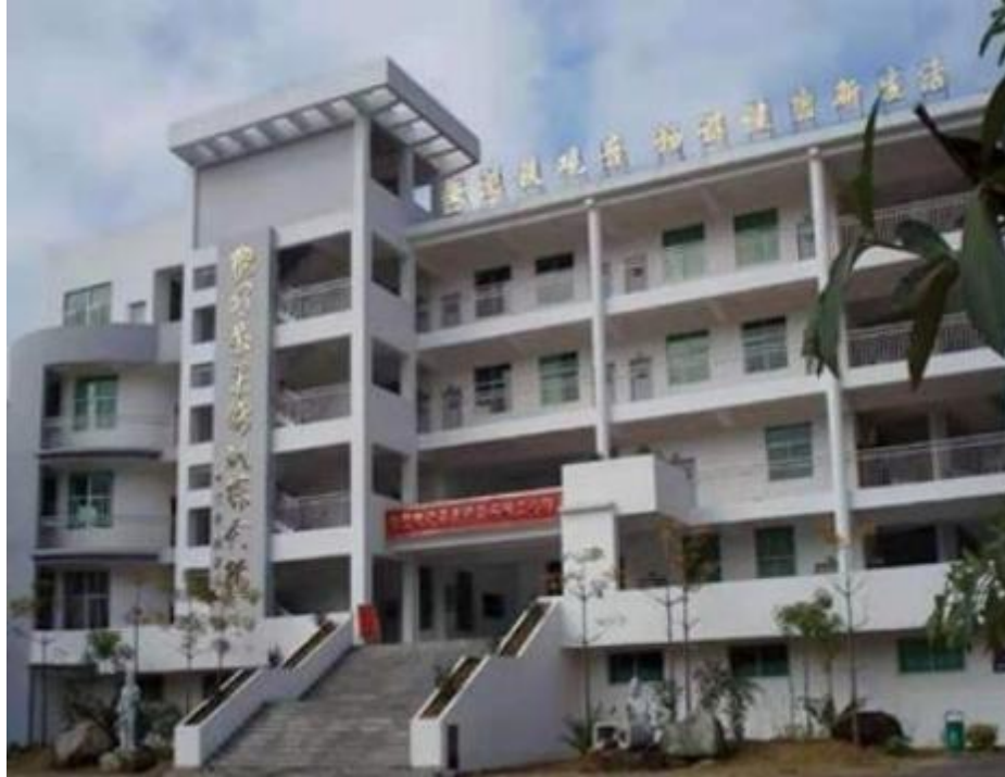
Photo 48 Tea Technology Complex Building in Anxi Vocational and Technical School of Tea
