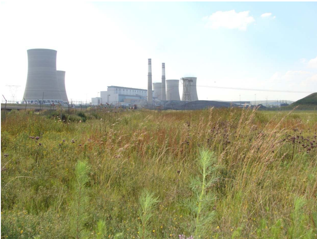
Route D & F looking in a northern direction in the temporary wetland zone.
