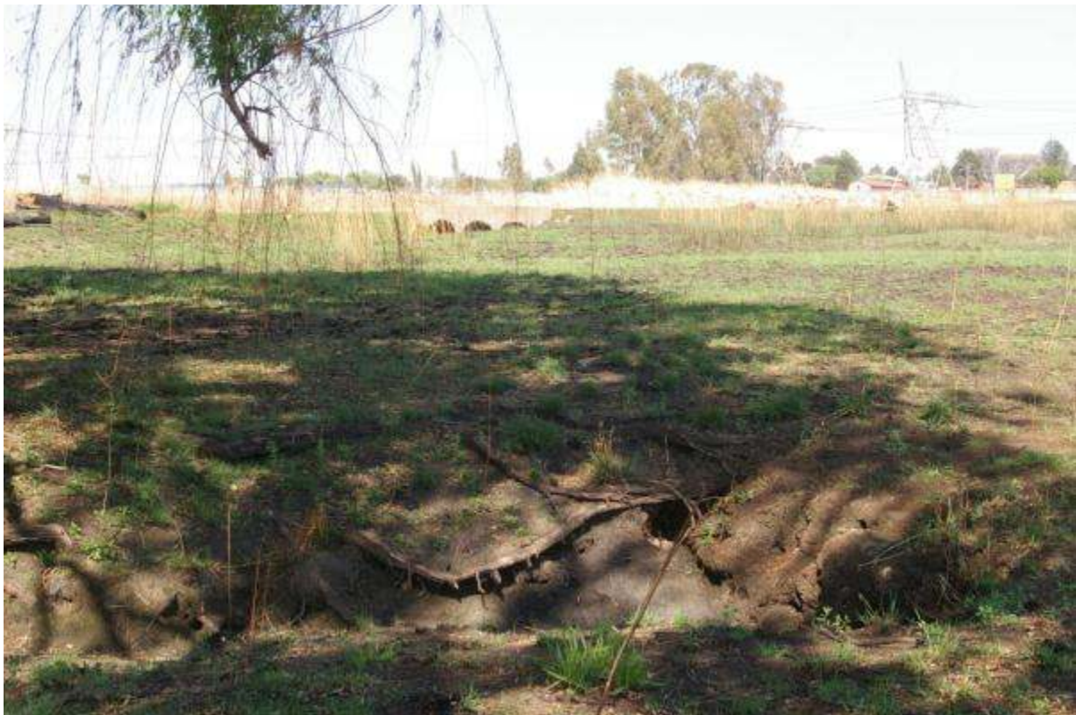
Figure 19. Erosion in the channel of the northern wetland unit. (Alternative 4)
