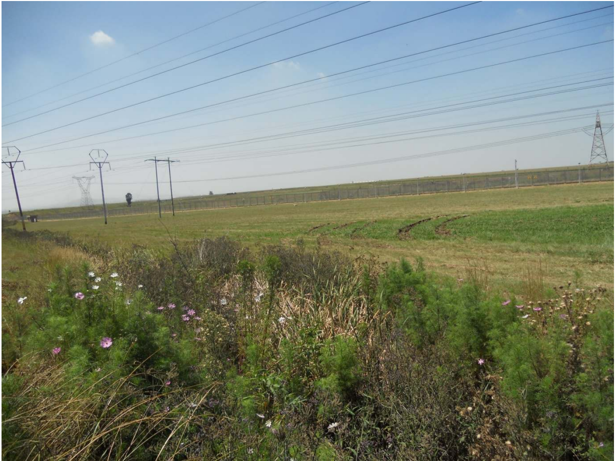
Figure 9. Artificial wetland present inside the power station fence.
