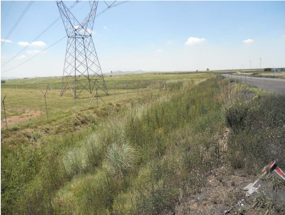
Alternative D, between dam and road. Looking in southern direction, close to turn to the west.
