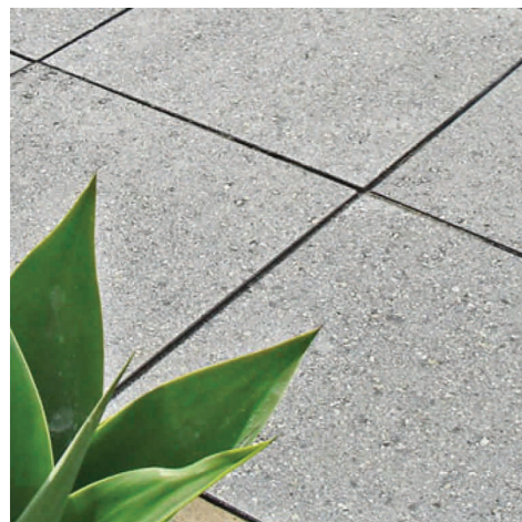
CONCRETE PAVERS (COURTYARD) Supported on pedestal and framing system
