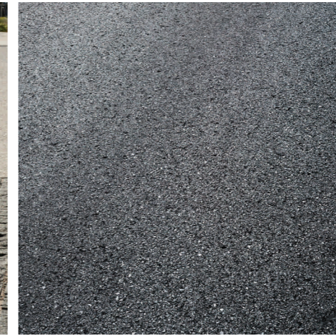
ASPHALT Carriage way/ Car Park
