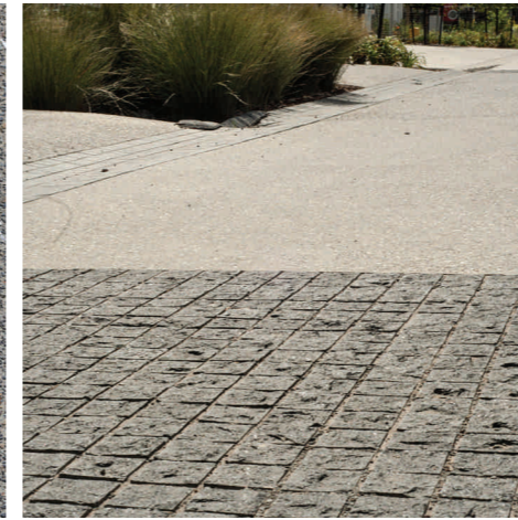
CROPPED SETTS Carriageway paving banding
