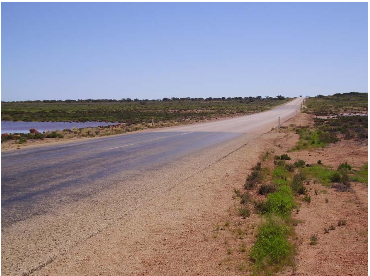
Photograph 6. 25.23 SLK – Minilya Exmouth Road. Lyndon River Crossing. RHS. North View.
