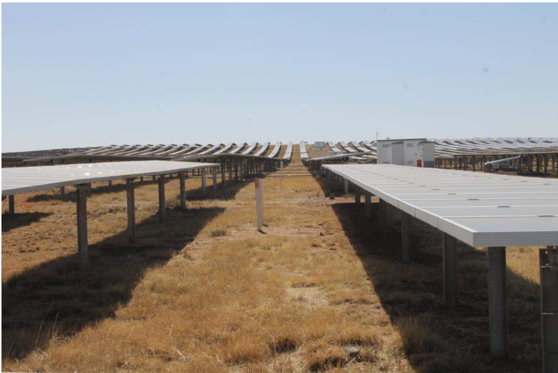
Figure 11. Image of solar arrays indicating the limited influence that such structures generally have on the flow of surface waters within a solar facility.
