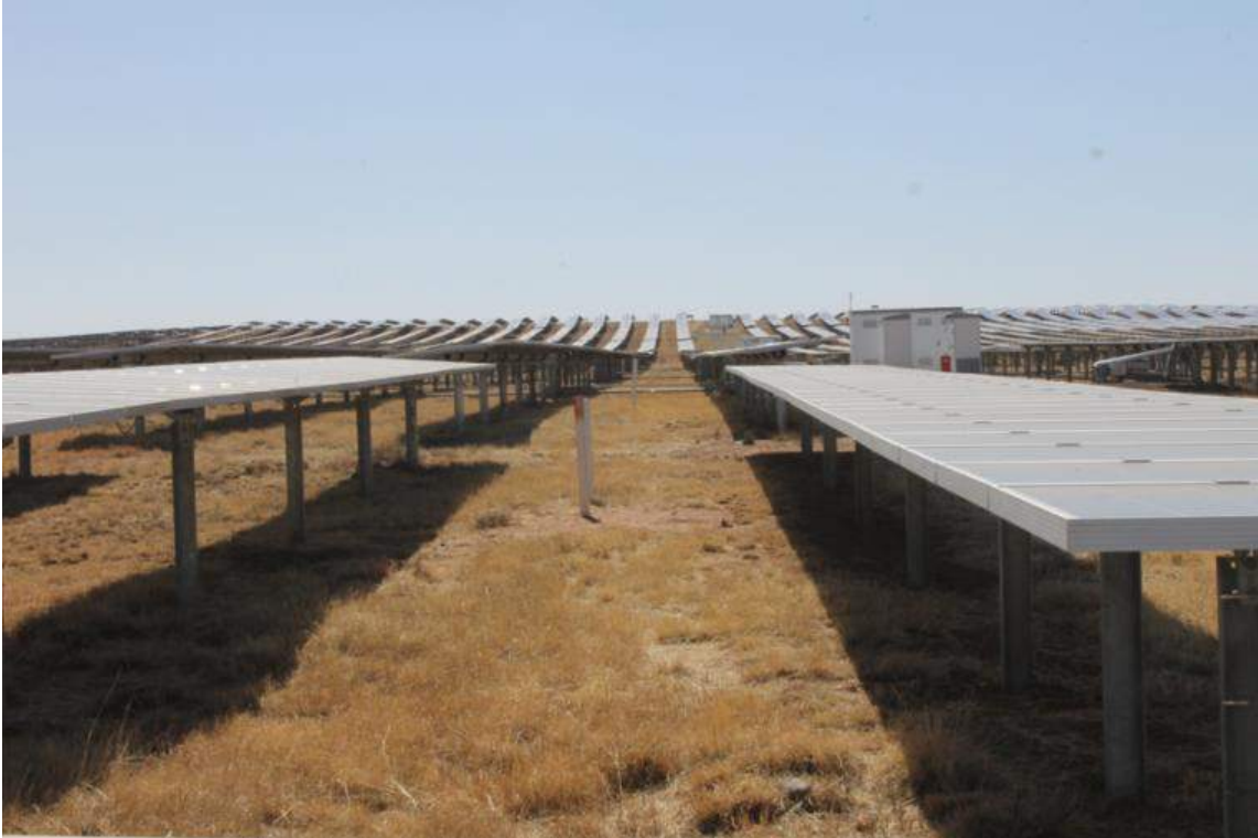
Fig. 13. Image of solar arrays indicating the limited influence that such structures generally have on the flow of surface waters within a solar facility.
