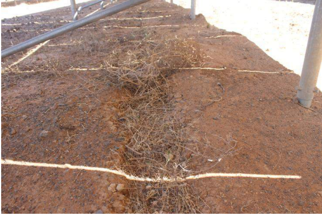
Figure 22. Image indicating rilling and plant invasion in rill under PV module. Habitat form and structure will change on site as a consequence of the establishment of PV modules
