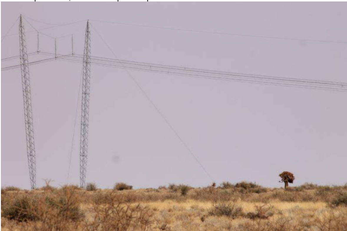
Figure 7 Image showing existing powerline near Skeerhok Alternative 1, with A dichotoma present in close proximity to tower.
