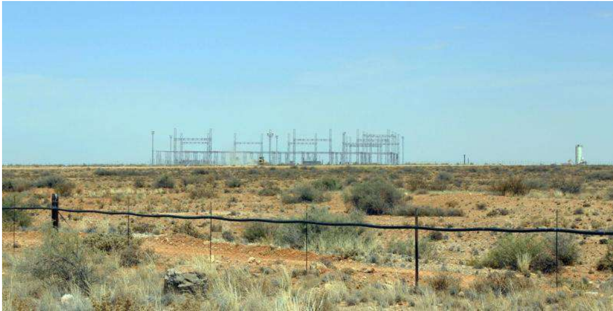
Figure 6: Photograph depicting the Eskom Nieuwehoop substation under construction (CSIR, 2016a; photo credit: Henry Holland).
