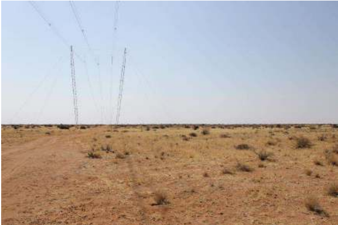
Figure 6: Image indicating the general nature of Skeerhok Powerline Alternative 1. Note existing powerline, which will in part run parallel to the Skeerhok Powerline Alternative 1
