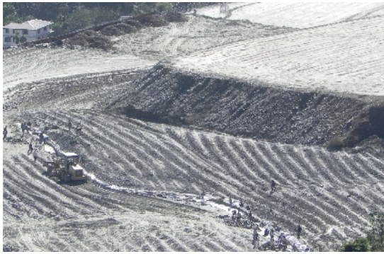
Damage due to deforestation and urbanisation
