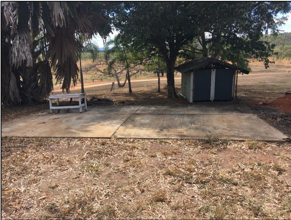
Figure 7 This large concrete pad could accommodate two air-conditioned shipping containers that could be used for seed storage.
