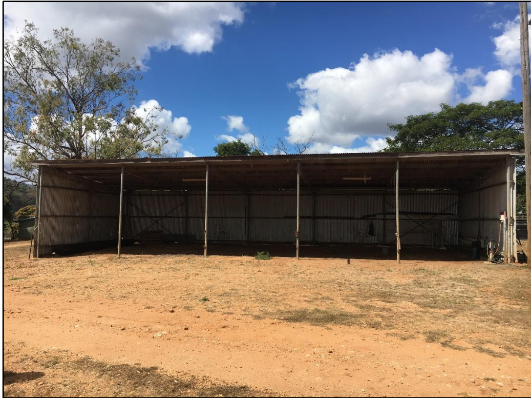
Figure 4. The five bay shed would require a concrete base and enclosed before considering it for seed drying or storage area.
