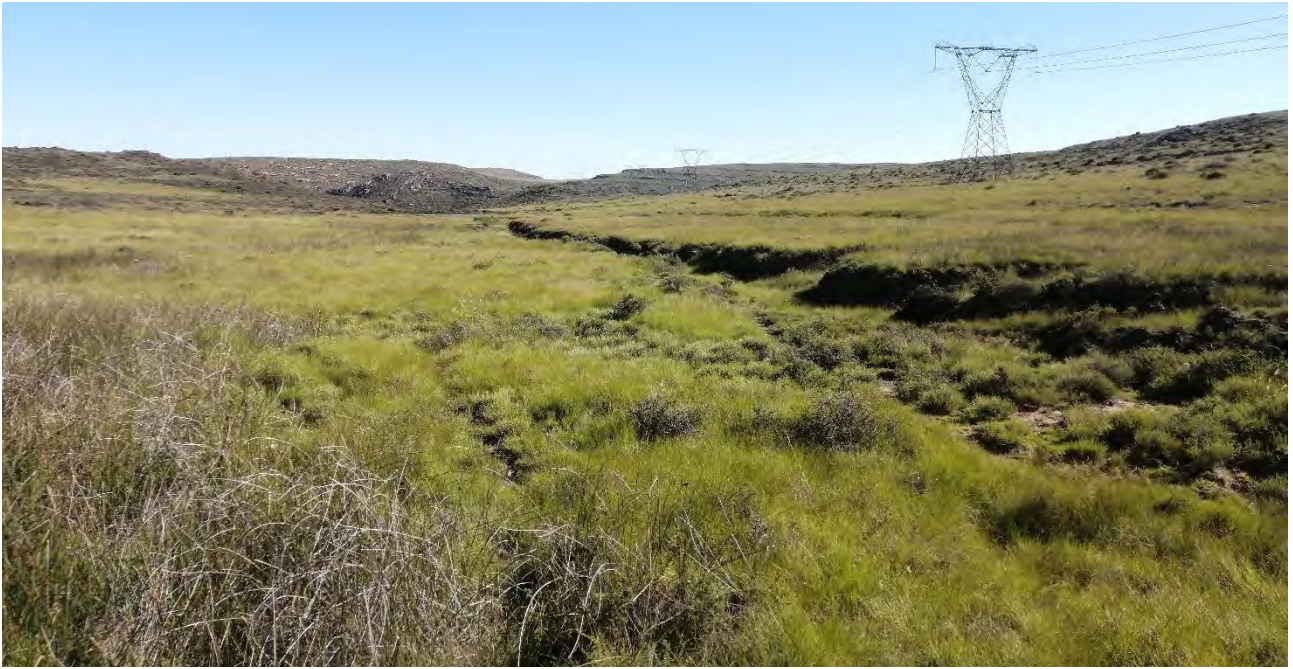
Plate 3.4: Erosion along a drainage line within the project area.
