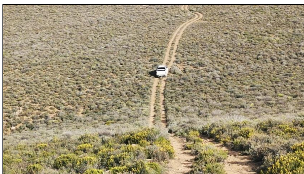
Figure 75: Typical two-track type farm road.
