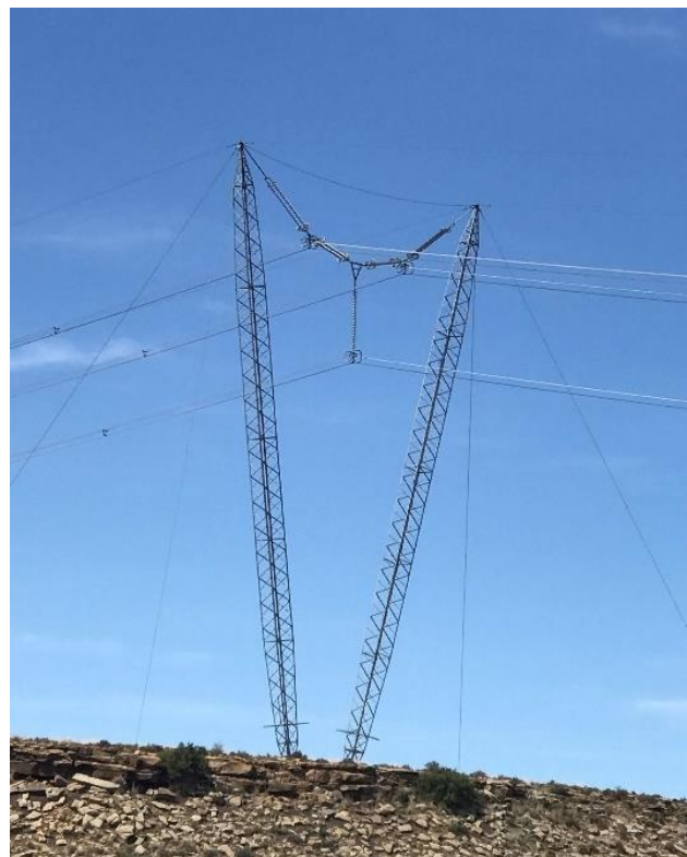
Figure 79: Pylon design that provide fewer opportunities for nesting sites.
