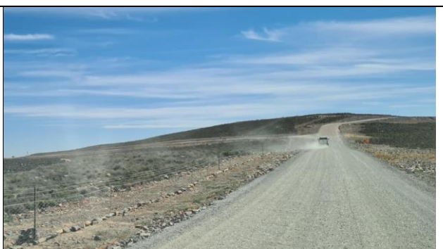
Figure 76: Typical WEF constructed access road.
