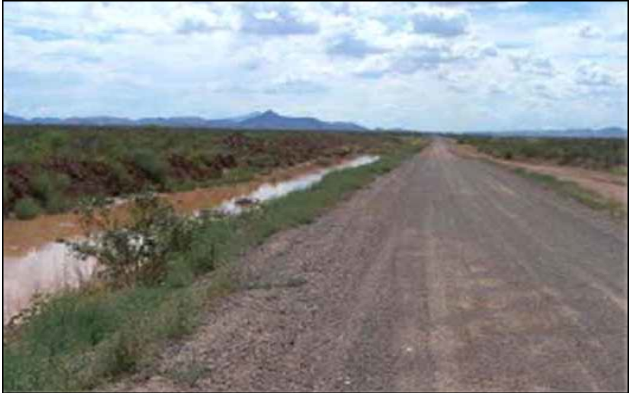
Figure C-3. FC-2 All-Weather Road (Photograph)
