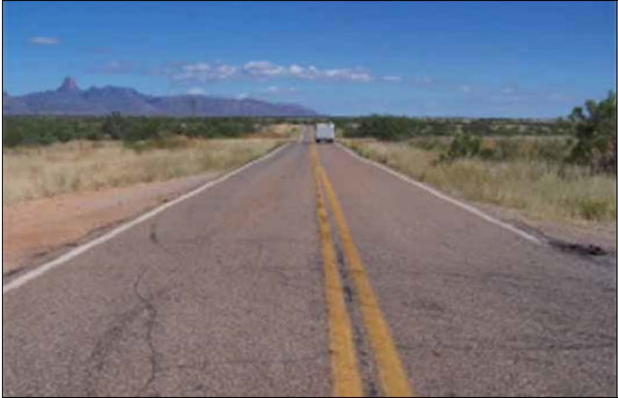
Figure C-1. FC-1 Paved Road (Photograph)
