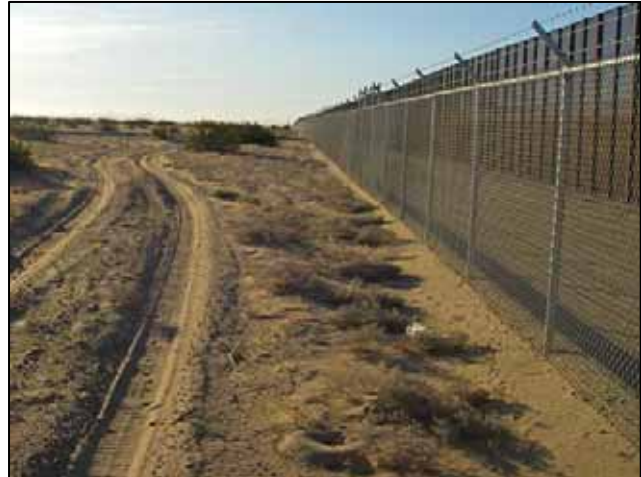
Photograph 2-2. Junction of Avenue D and USBP BIS, facing east.
