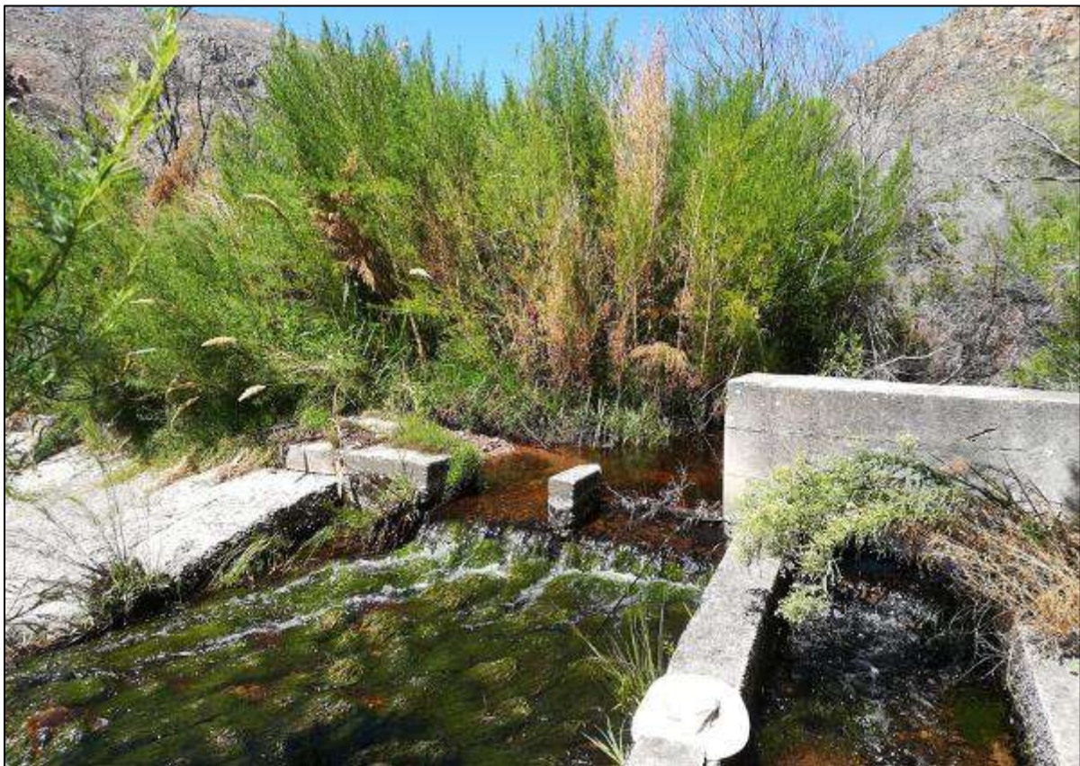
Figure 5.2: Weir on the Boesmans River, with a lot of water being diverted into the canal visible in the right-hand corner. Photo: Jeanne Gouws.
