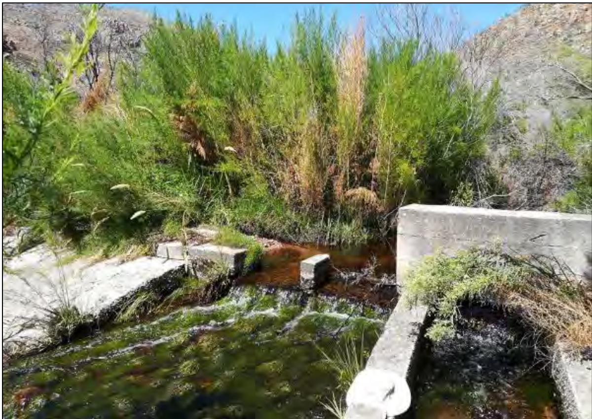
Figure 5.2: Weir on the Boesmans River, with a lot of water being diverted into the canal visible in the right-hand corner. Photo: Jeanne Gouws.
